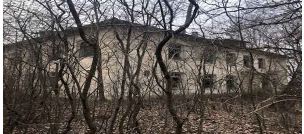
Picture 1: Current situation of the construction in Dashava
